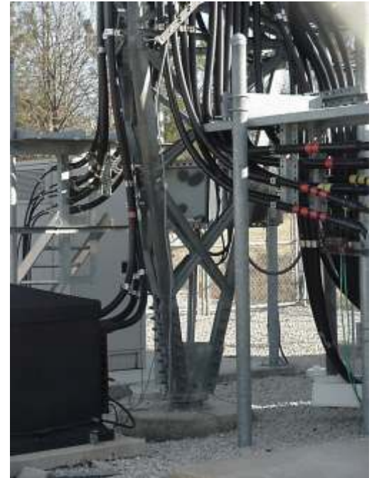
CES Towers feature an articulated base for stress free tower alignment Problematic anchor bolts are not necessary.
